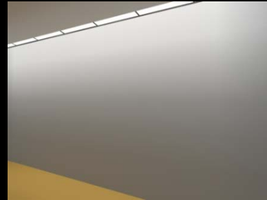
#2 Semi-recessed linear fluorescent wall-washer
