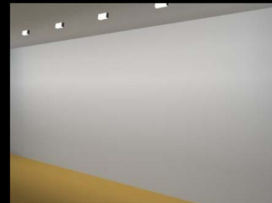
#3 Semi-recessed metal Halide wall-washer
